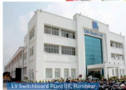
LV Switchboard Plant (II), Haridwar
