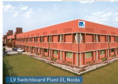
LV Switchboard Plant (I), Noida
