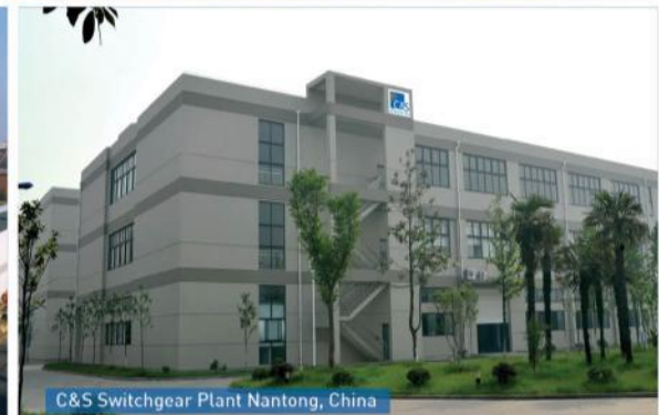
C&S Switchgear Plant Nantong, China
